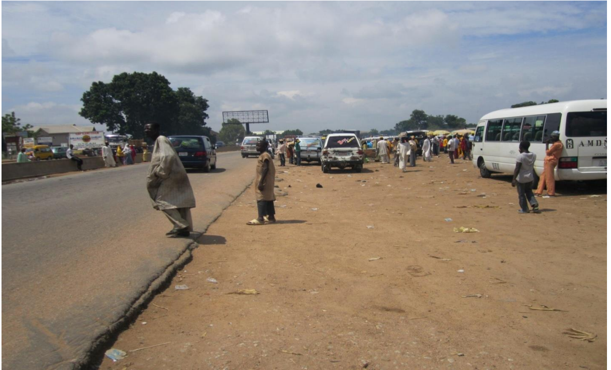
Picture 14 (P14) Improper bus stop location close to the road km 6+800
