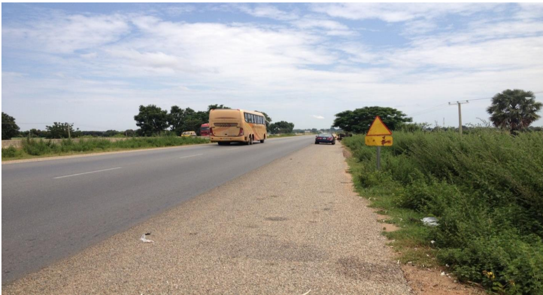
Figure 4.5 Worn Out Sign (Km 5+300)
