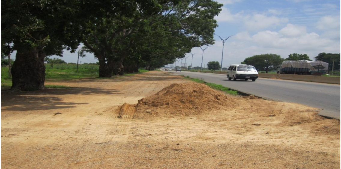
Figure 4.4 Dangerous Trees within the Safety Zone Area (Km 13+100)
