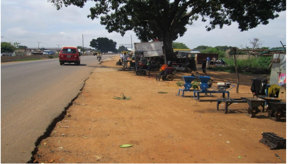
Picture 13 (P13) Dangerous tree and objects close to the road km 17+600
