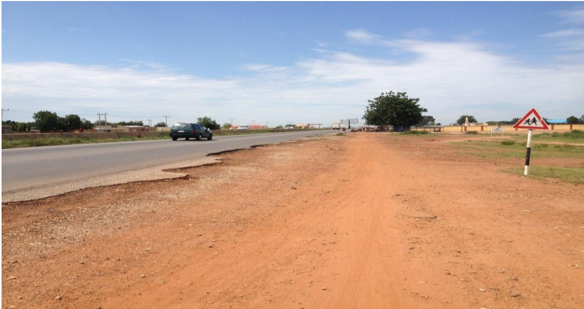
Figure 4.7 Improper Pedestrian Crossings (Km 5+200)
