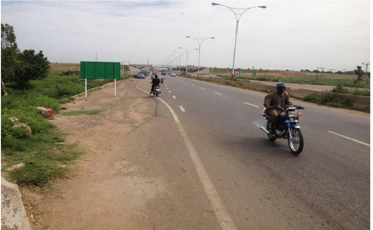
Picture 16 (P16) Dangerous road narrowing km 0+300
