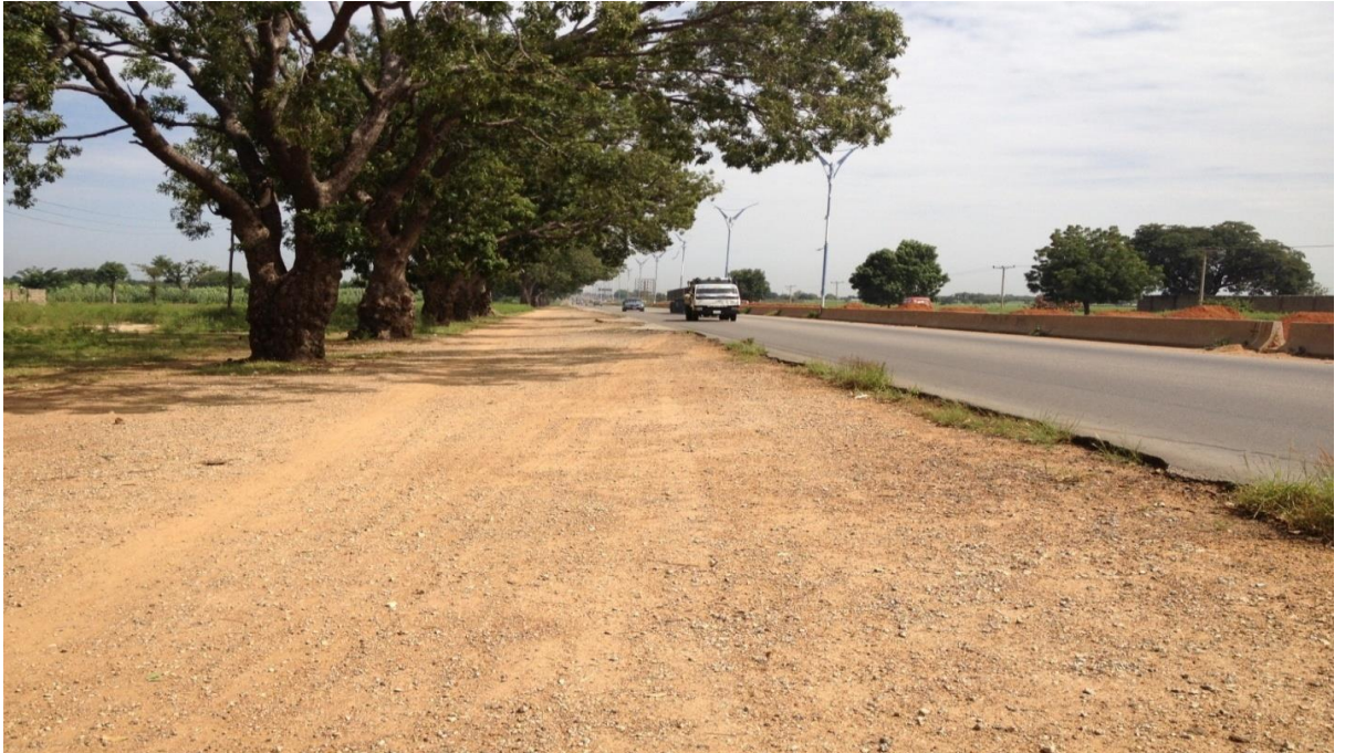
Picture 3 (P3) Dangerous trees within the safety zone area km 16+500
