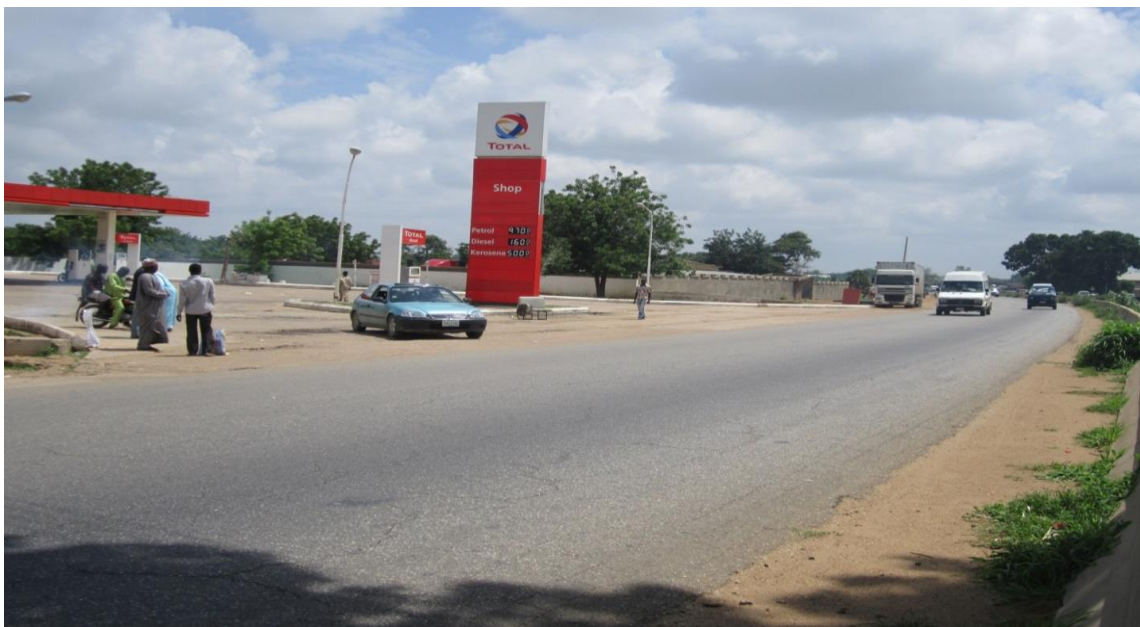
Figure 4.6 Improper Connection to Gas Station (Km 3+400)
