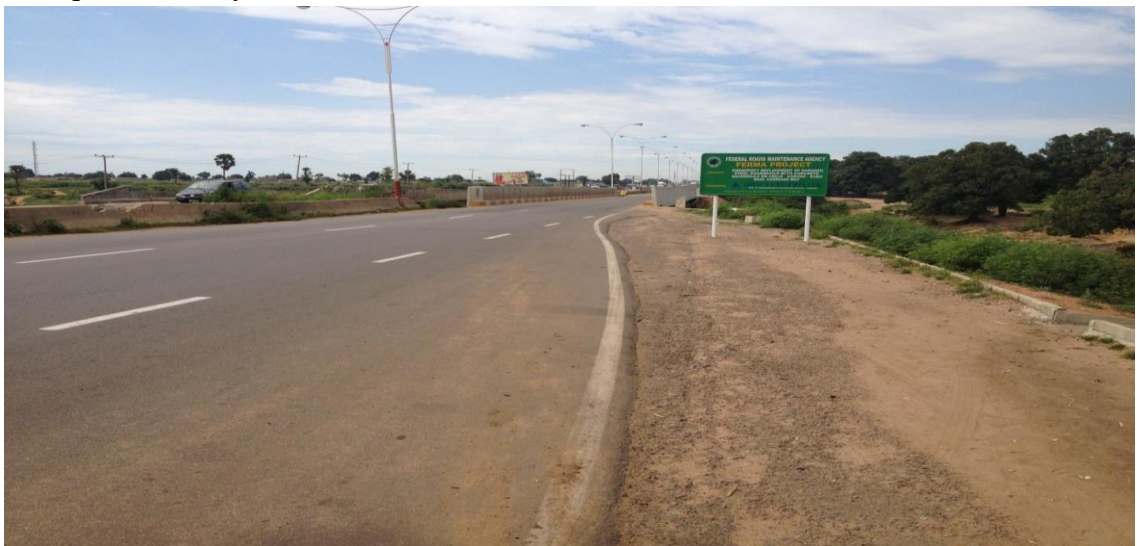
Figure 4.15 Dangerous Road Narrowing (Km 0+300)
