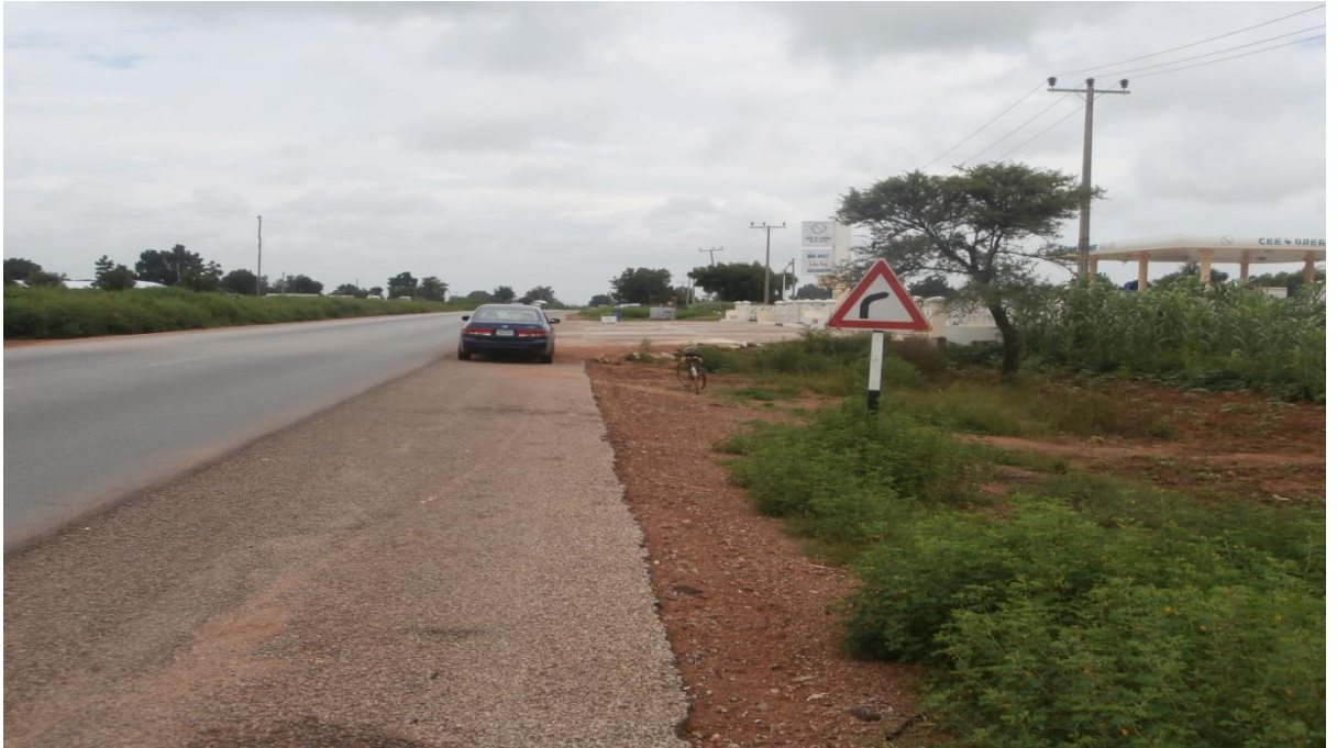
Picture 23 (P23) Limited sight distance km 16+200
