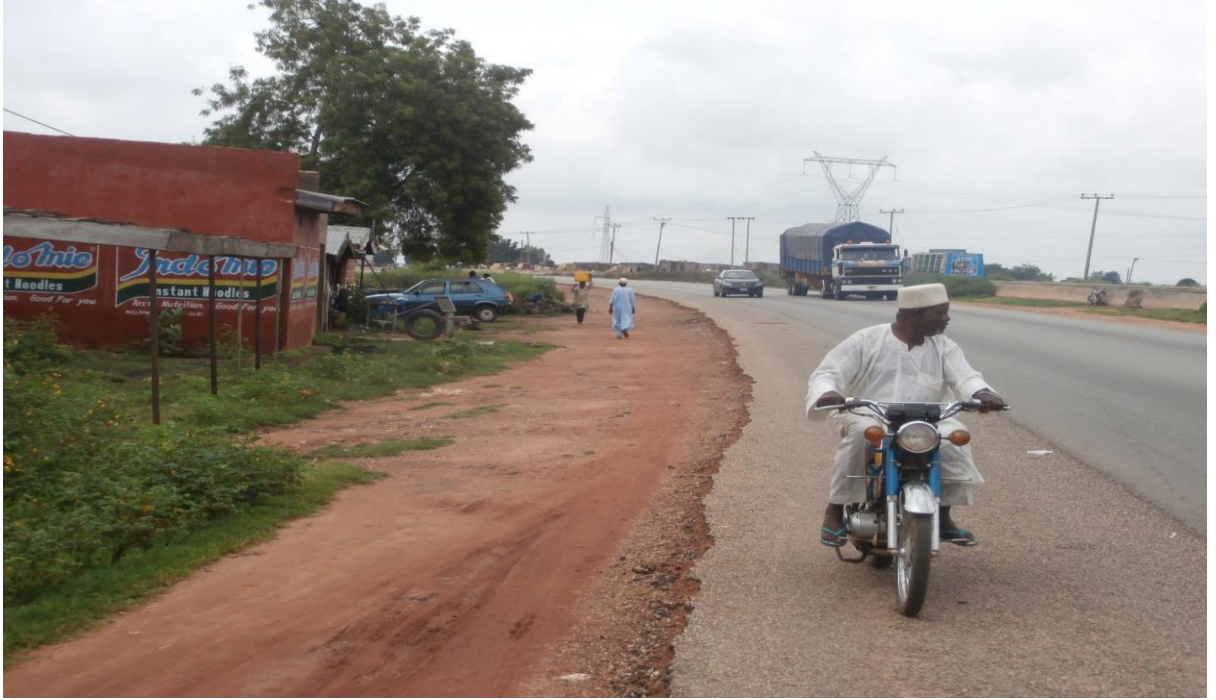
Picture 15 (P15) Dangerous house within the safety zone km 38+700
