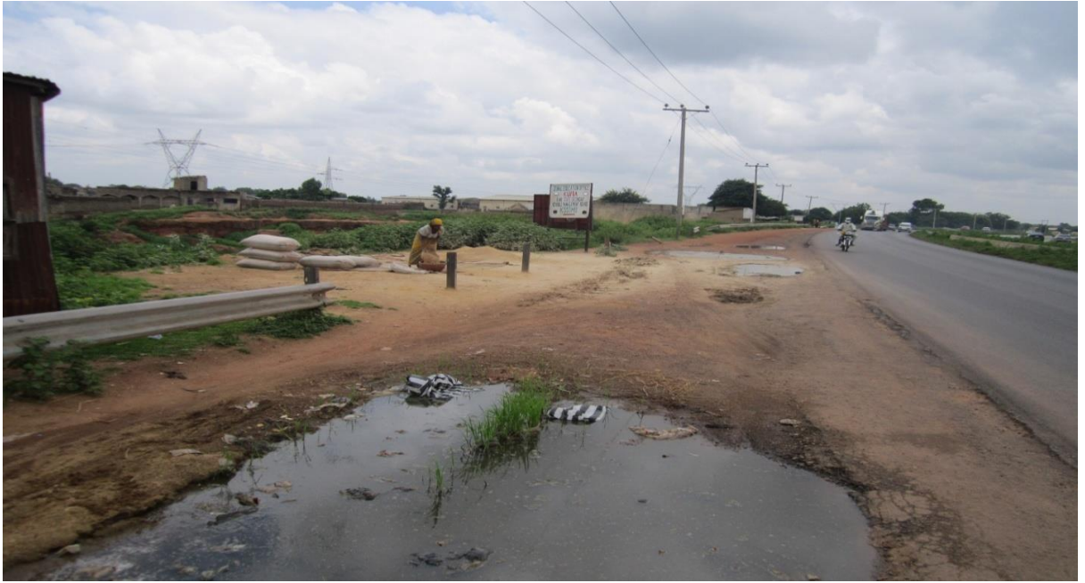
Picture 11 (P11) Dangerous guardrail section km 21+500
