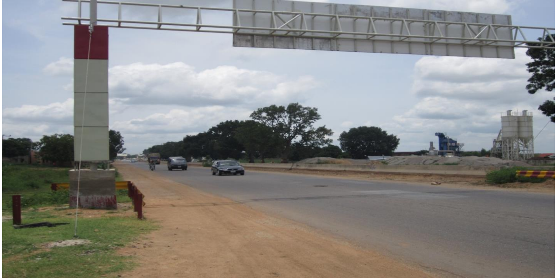
Figure 4.14 Dangerous Concrete for Support Close To the Road (43+200)
