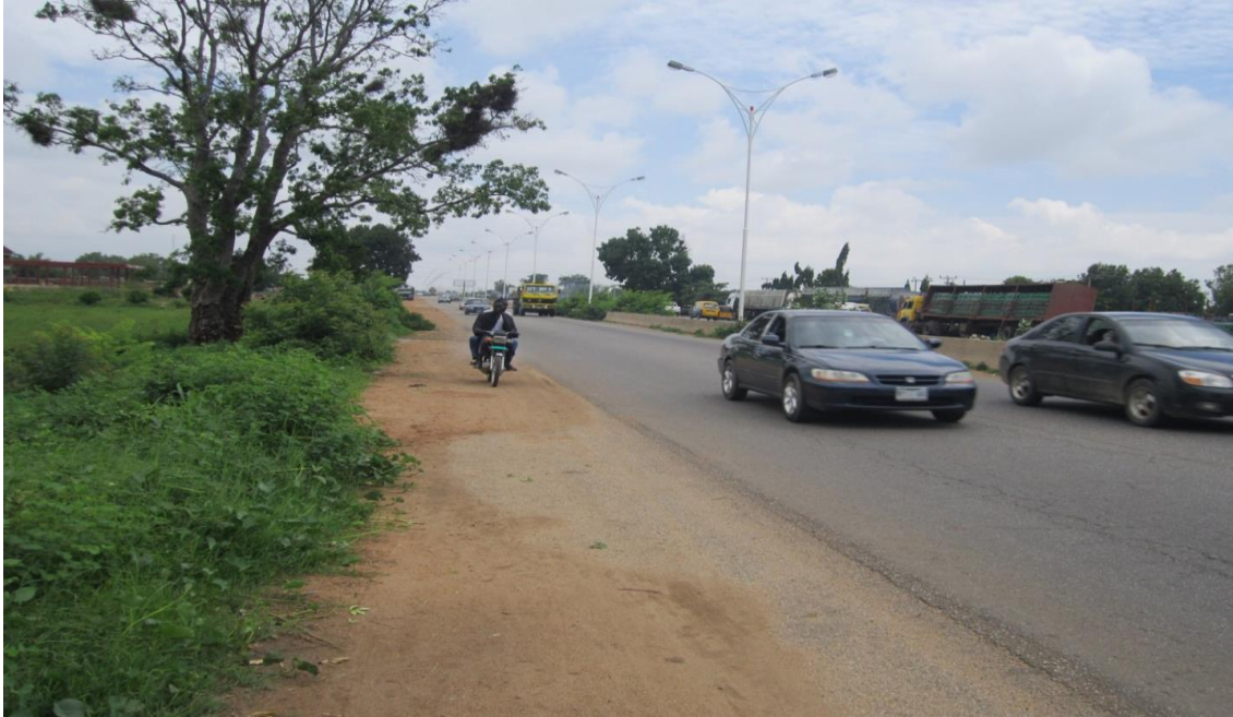
Figure 4.16 Missing Safety Zone (Km 5+900)
