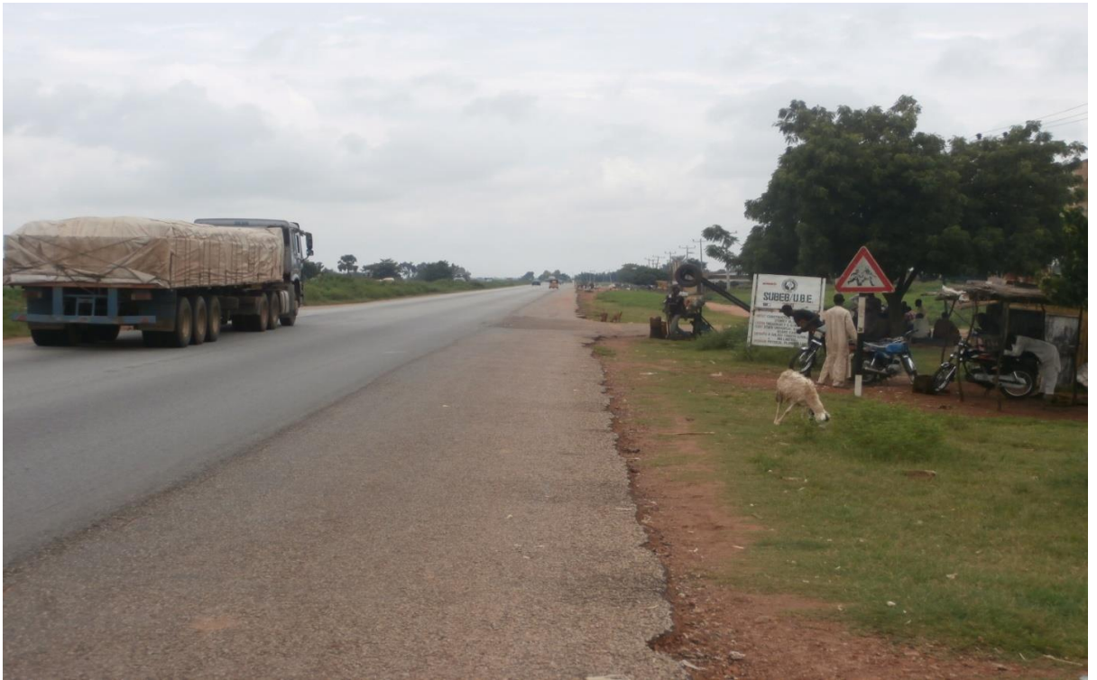
Picture 8 (P8) Improper pedestrian crossing km 41+300
