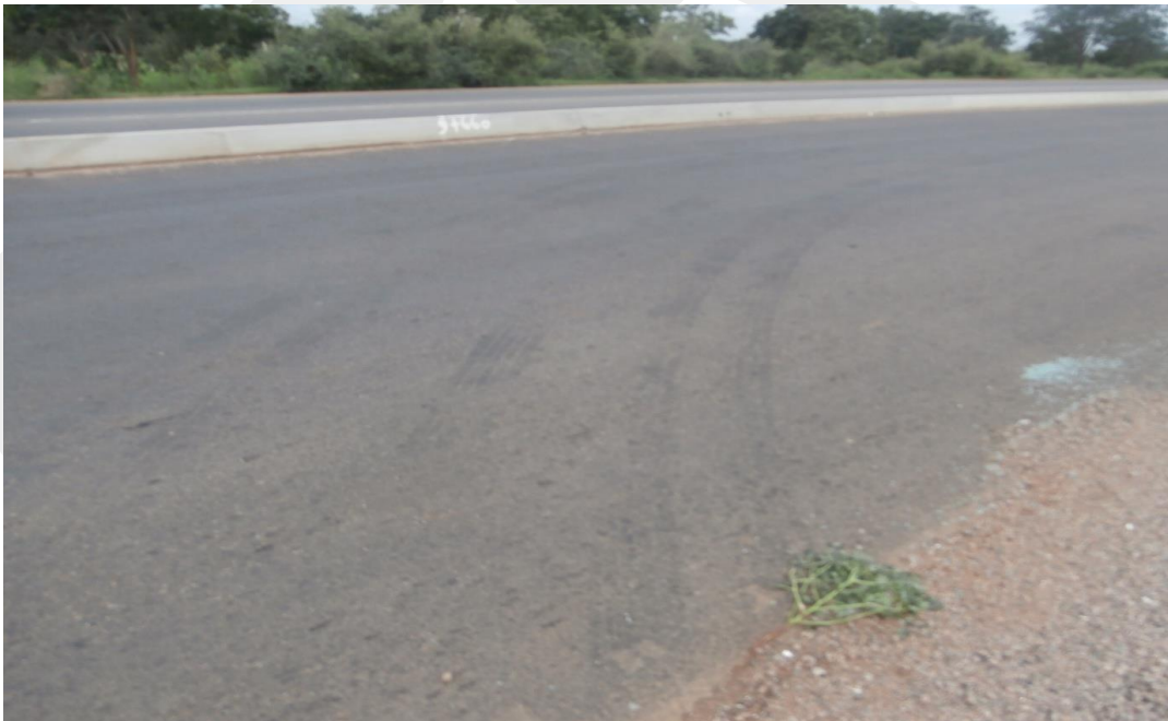
PICTURE SHOWING SKID MARKING PRODUCE BY THE INVOLVED BUS
