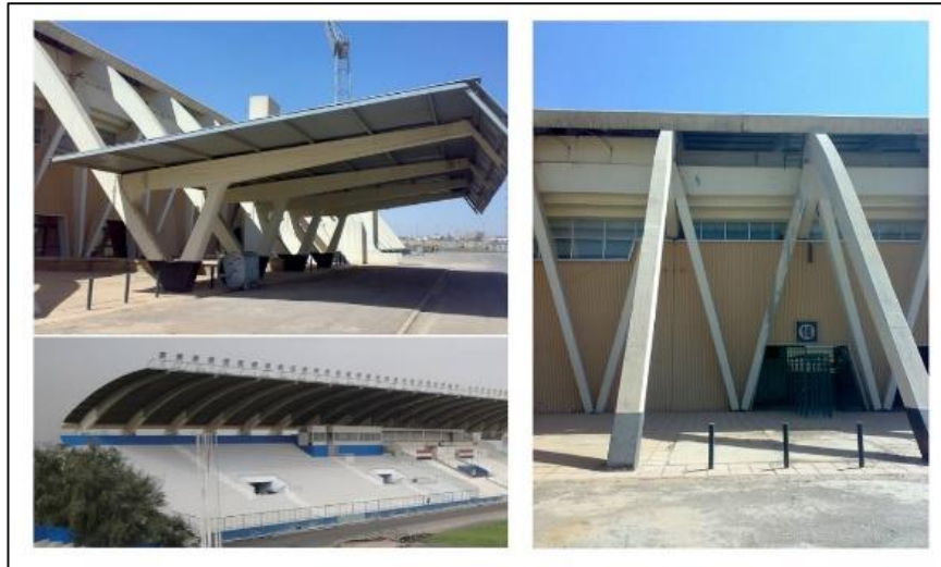
Figure 2. 2 Real photos for the structure of the straight-line stands cover. (Photo by the author Abdullah Allawi)
