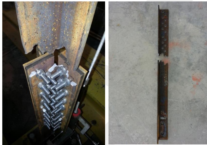
Figure 2.71. Rupture on critical path of Specimen-5
