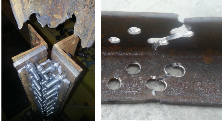
Figure 2.95. Rupture on critical path of Specimen-7
