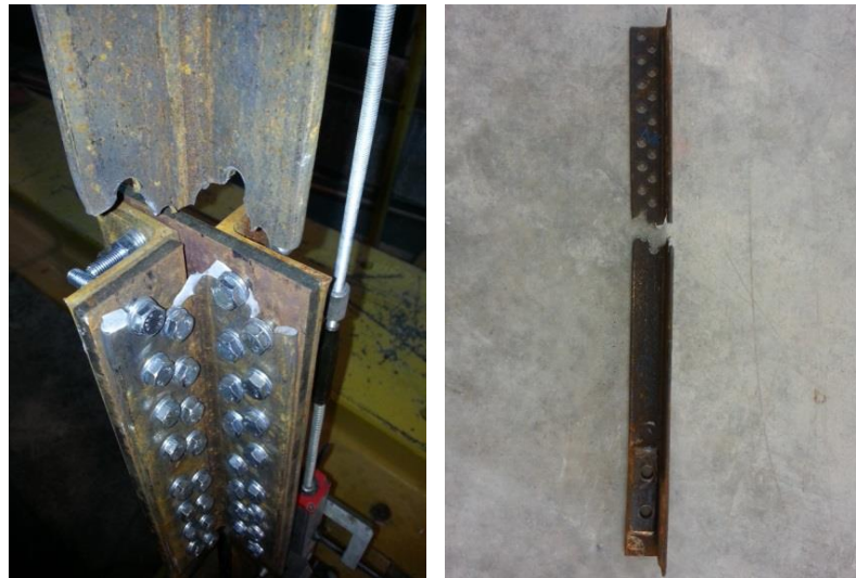
Figure 2.83. Rupture on critical path of Specimen-6
