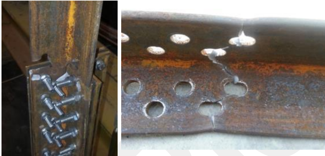
Figure 2.49. Rupture on critical path of Specimen-3
