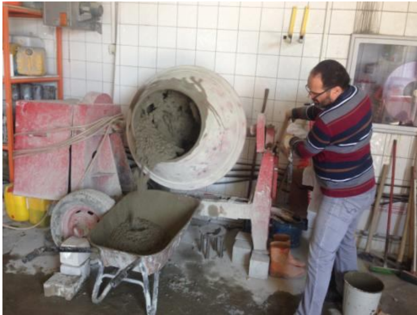
Figure 3-7 – Mixing of materials
