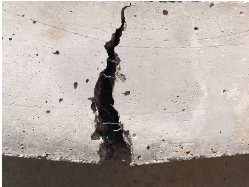
Figure 4-5 – Typical failure mode of SFRC prisms under flexure
