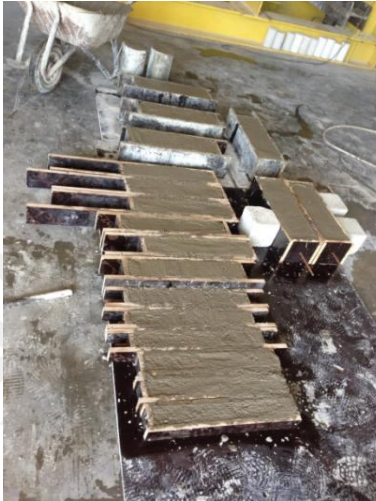
Figure 3-9 – Placing concrete into molds and formworks
