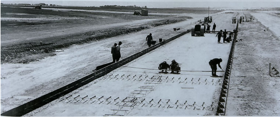
Figure 3. The construction of the reinforced concrete runway at Yeşilköy Airport, with its transverse and longitudinal steel supports, general view, c.1950. Sarıgöl, op. cit., p. 103 (used with permission).
