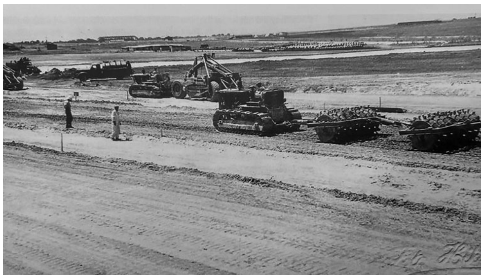
Figure 2. Soil compaction of the reinforced concrete runway at Yeşilköy Airport, c.1950. Sarıgöl, op. cit., p. 104 (used with permission).
