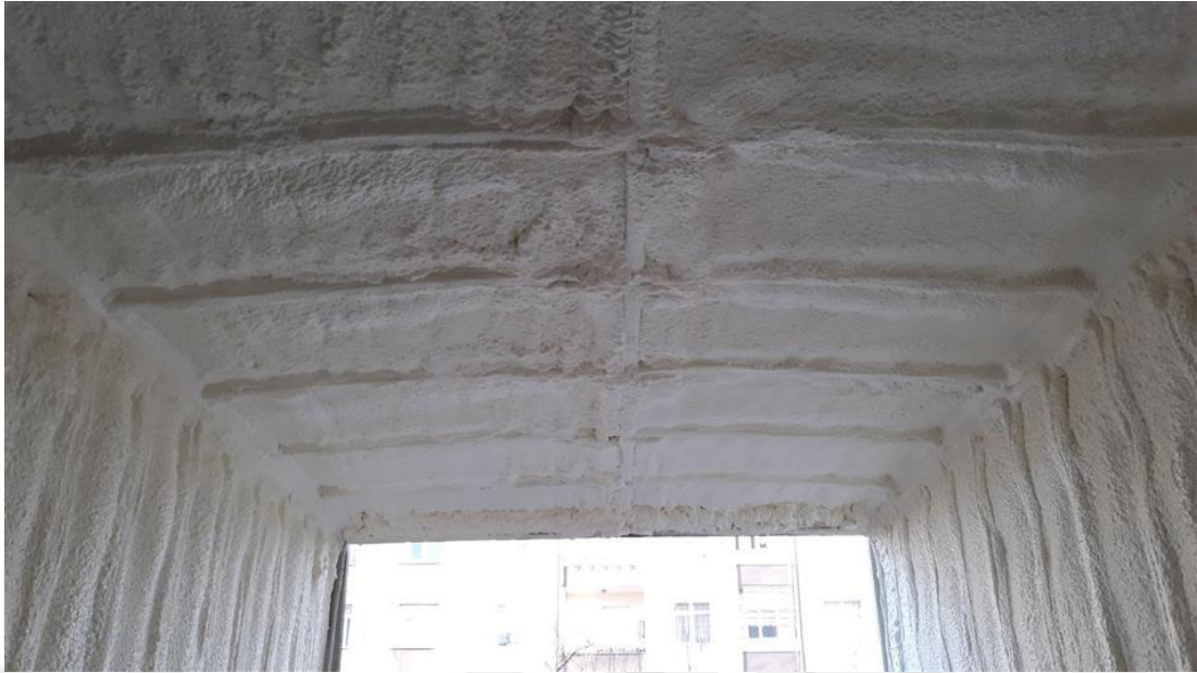
Figure 3.6 Polyurethane Foam Application [30].
