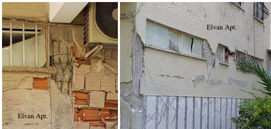
Figure 39. Short column formation in a severely damaged building
