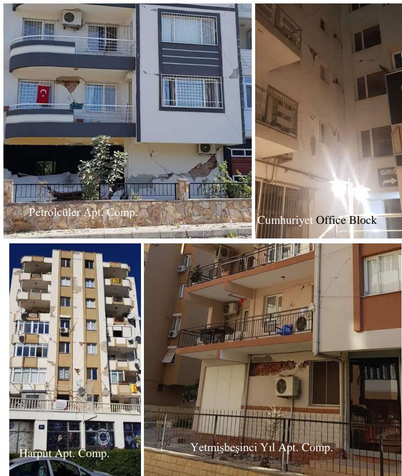
Figure 29. Diagonal cracks on structural and non-structural elements
