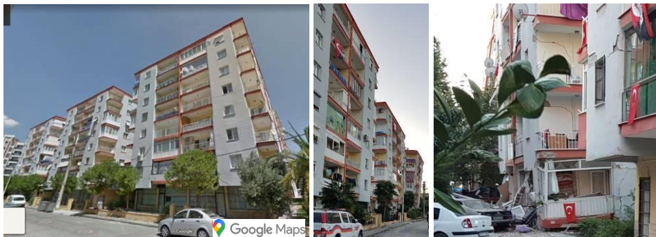
Figure 28. Photographs of the Cumhuriyet Apartment Complex before and after the earthquake
