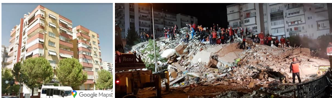
Figure 23. Photographs of the Emrah Apartment Building before and after the earthquake
