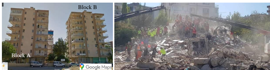
3 4 5 Figure 24. Photographs of Block B of the Yağcıoğlu Apartment Complex before and after the 6 earthquake
