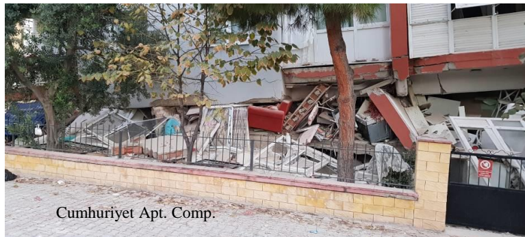
Figure 38. Collapsed buildings due to the failure of first story columns
