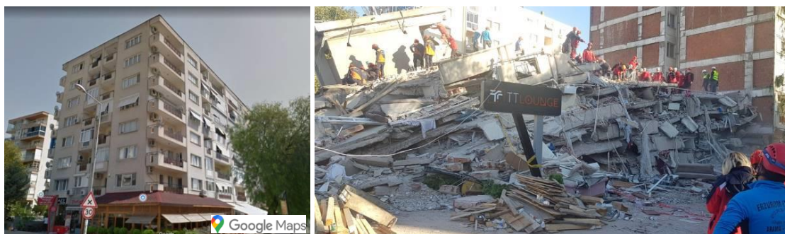
Figure 22. Photographs of the Doğanlar Apartment Building before and after the earthquake
