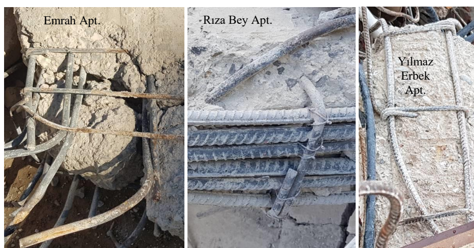
20 Figure 34. Reinforcement types in various collapsed buildings
