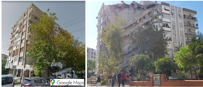
Figure 26. Photographs of the Karagül Apartment Building before and after the earthquake
