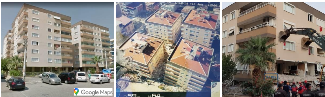
Figure 27. Photographs of the Barış Apartment Complex before and after the earthquake
