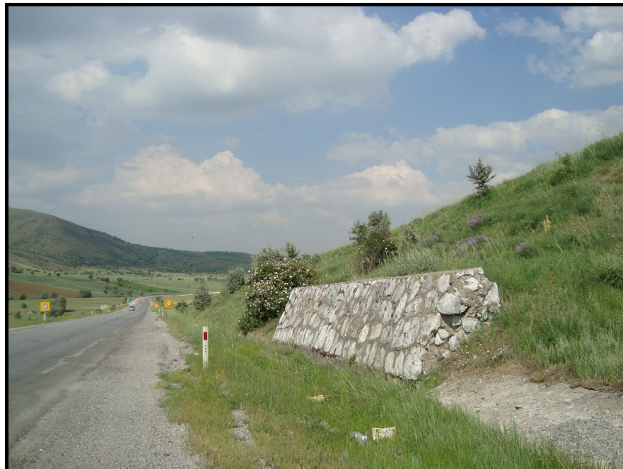
Figure 4.12 Shoulder missing
