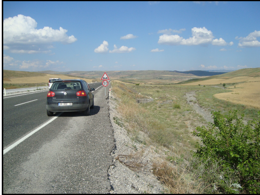
Figure 4.13 Improper sign usage in the shoulder zone
