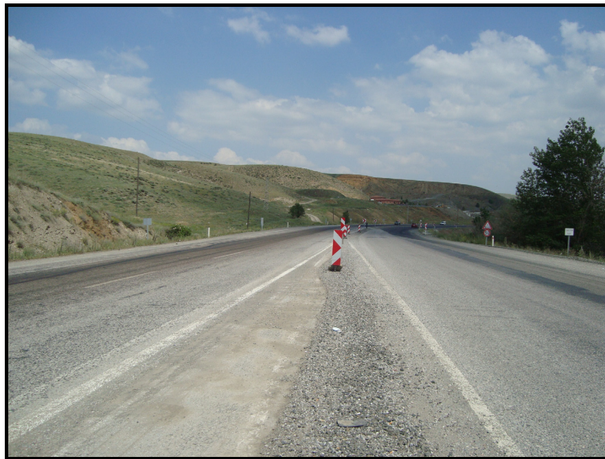
Figure 4.11 There is no ditch structure in the median zone
