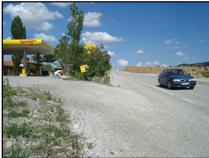
Figure 4.8 Dangerous exit section of gas station
