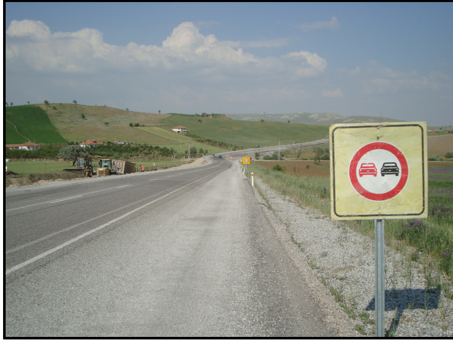
Figure 4.6 Improper sign usage
