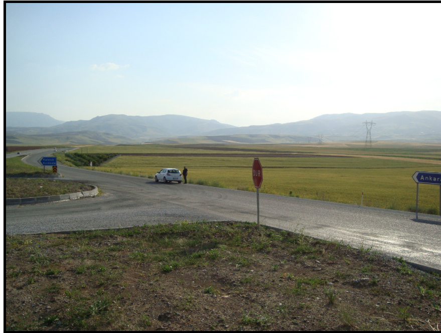
Figure 4.7 Improper junction design
