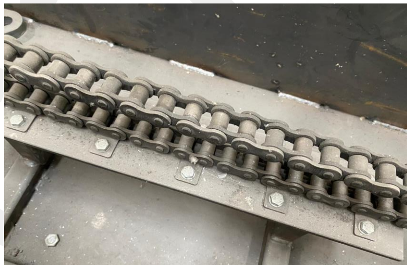
Figure 4.17: Fixing process of the chain.
