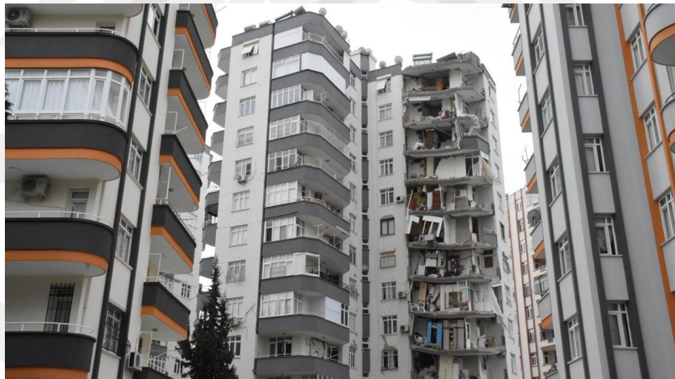
Figure 1.2 Damaged Building By Earthquake in Kahramanmaraş Province, TRTHABER [4]
