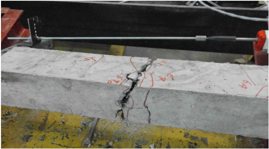
Figure 4-15 – Typical crack patterns for SFRC tension specimens (SFRC100×100×500-01)
