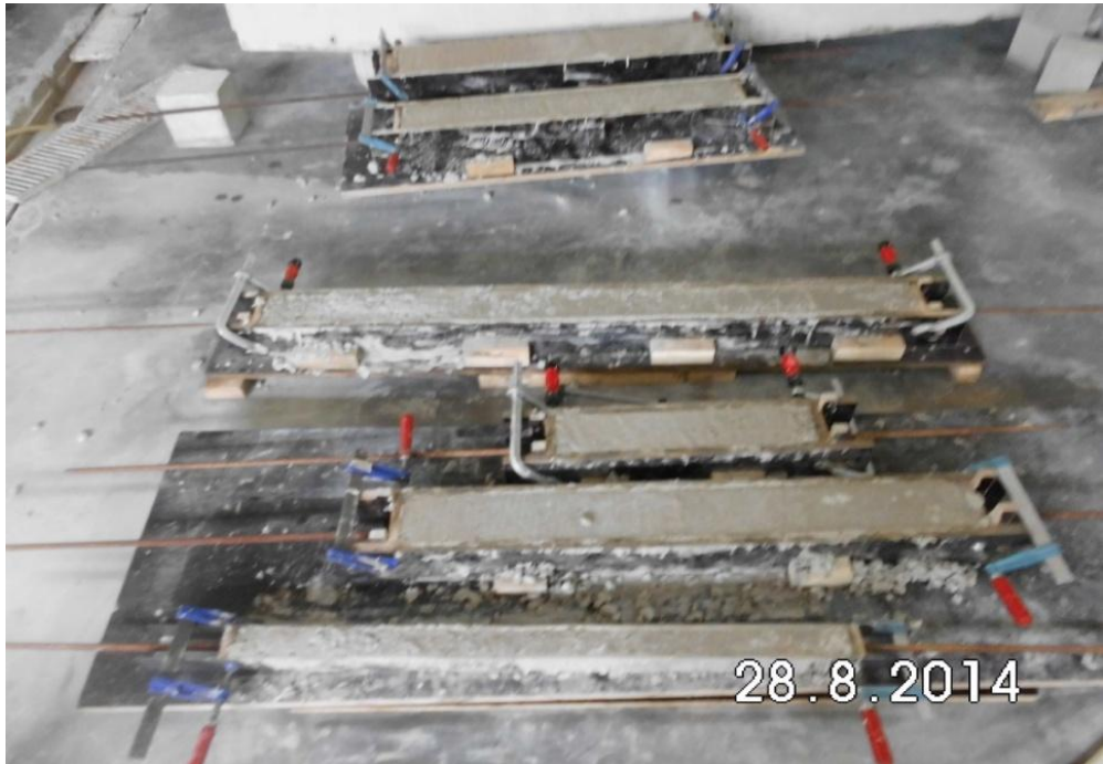
Figure 3-8 – Placing concrete in formwork
