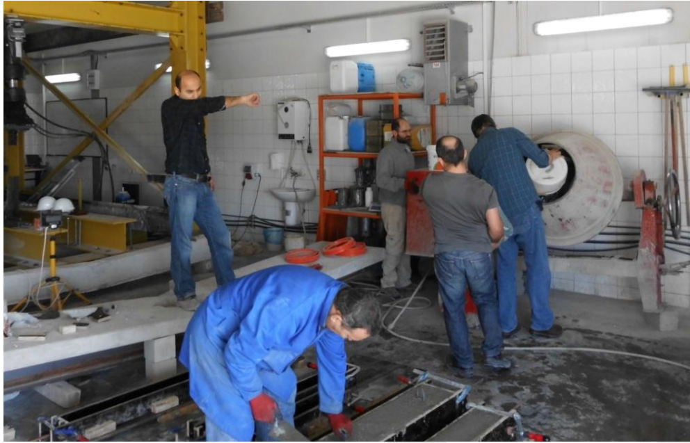
Figure 3-7 – Mixing of materials and placing concrete in formwork
