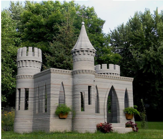
Figure 2.2: The world's first 3D printed castle printed in 2014 in The USA (Photo courtesy of Andrey Rudenko).
