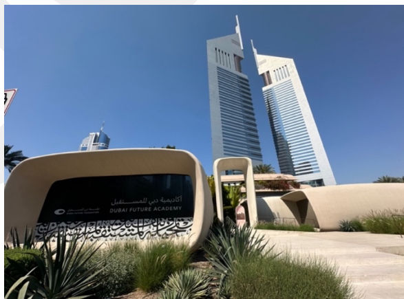
Figure 2.3: The world's first 3D printed office printed in 2016 in Dubai (Photo courtesy of Leva Latifiilkhechi).
