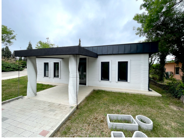
Figure 2.4: House printed in 2021 in Türkiye by İston Company (Photo courtesy of Saman Aminbakhsh).
