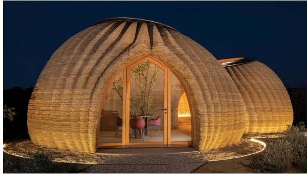
Figure 3.1: House printed houses in 2022 in Italy (Photo courtesy of Sarah Amelar).
