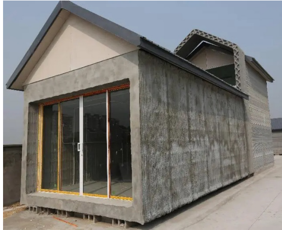
Figure 2.1: The world's first 3D printed house printed in 2014 in China (Photo courtesy of Karyne Levy).
