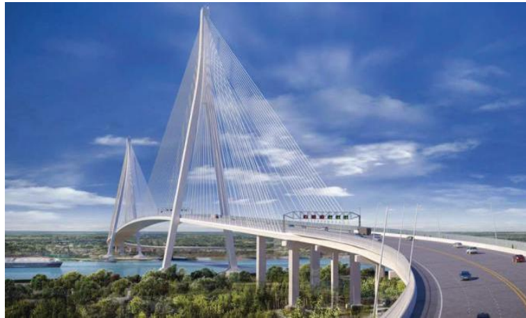
Figure 30 Gordie Howe International Bridge Project [84]
