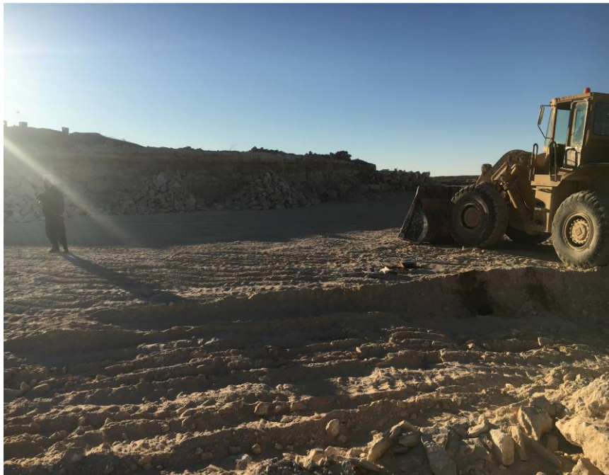
Figure 3.10 Collect and load rocks by an articulated loader
