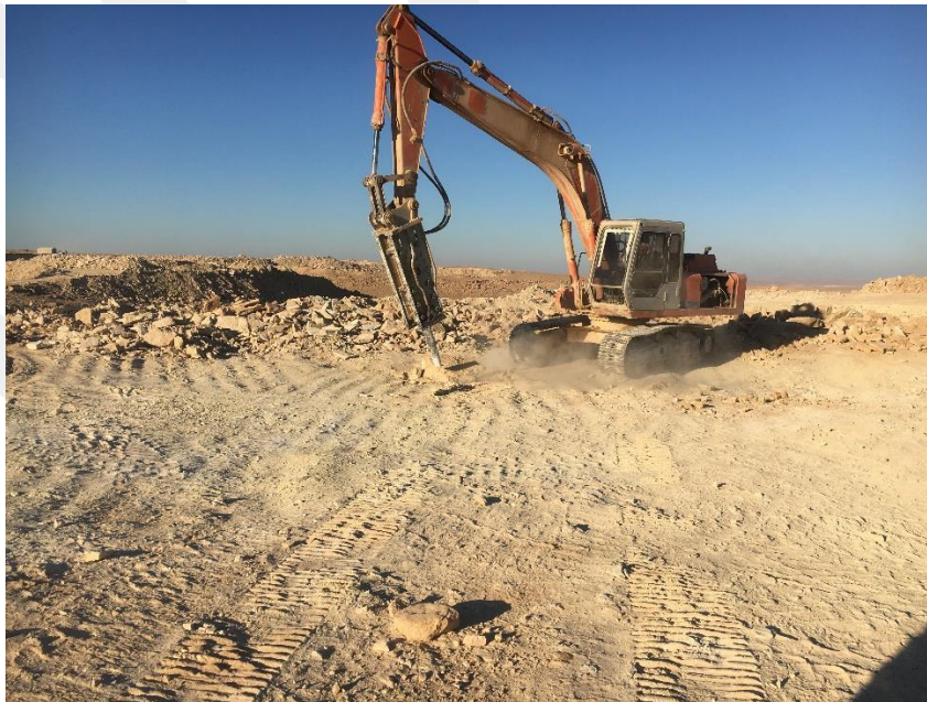
Figure 3.9 Hydraulic crushing hammer attached to an excavator
