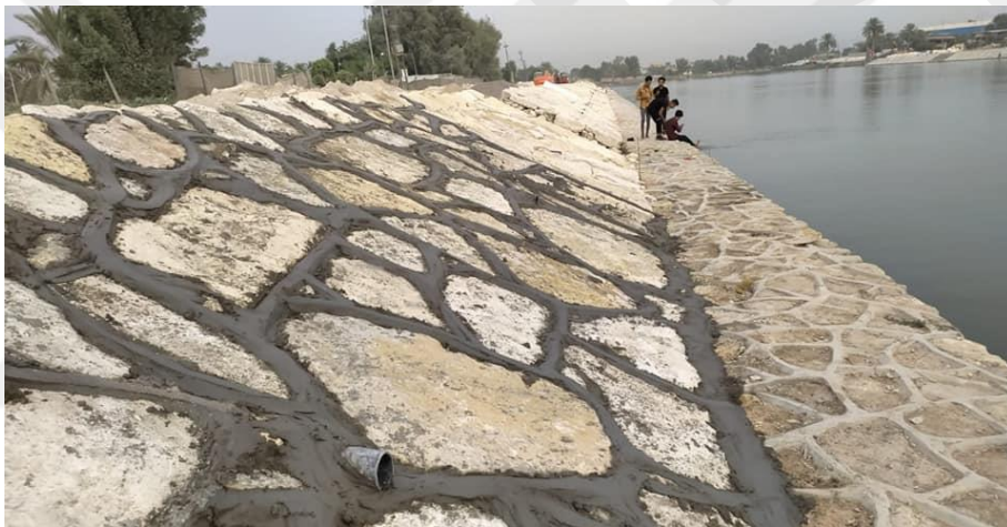
Figure 3.3 Cladding the banks of rivers and streams
