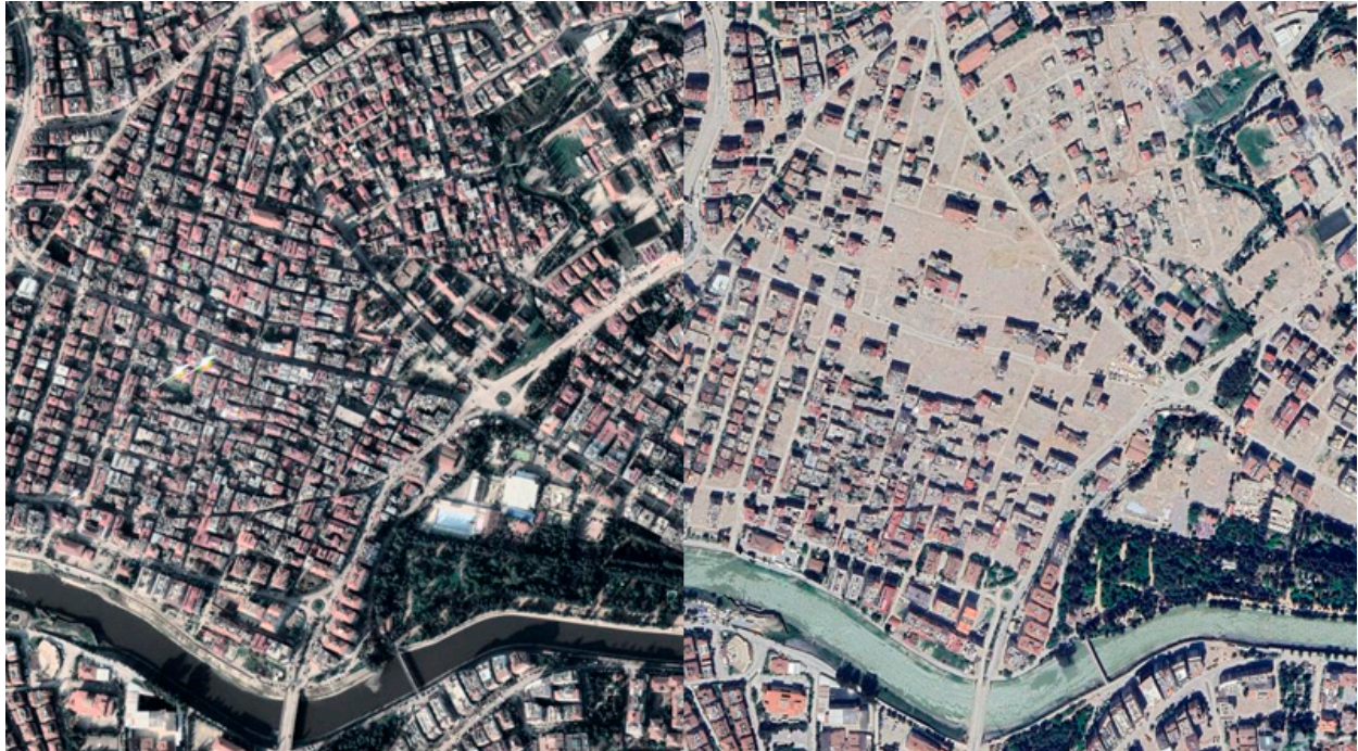
Figure 1. Satellite images before and after the earthquake in Hatay (taken from Google Satellite).
