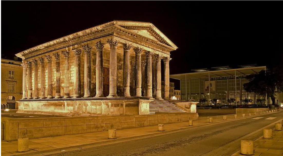
Figure 5 - Temple of Maison Carrée [2].
