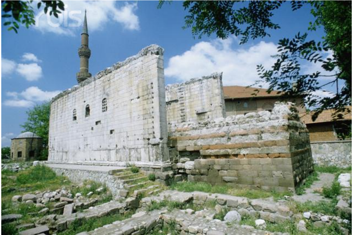
Figure 38 - Standing wall with foundation of Augustus Temple
