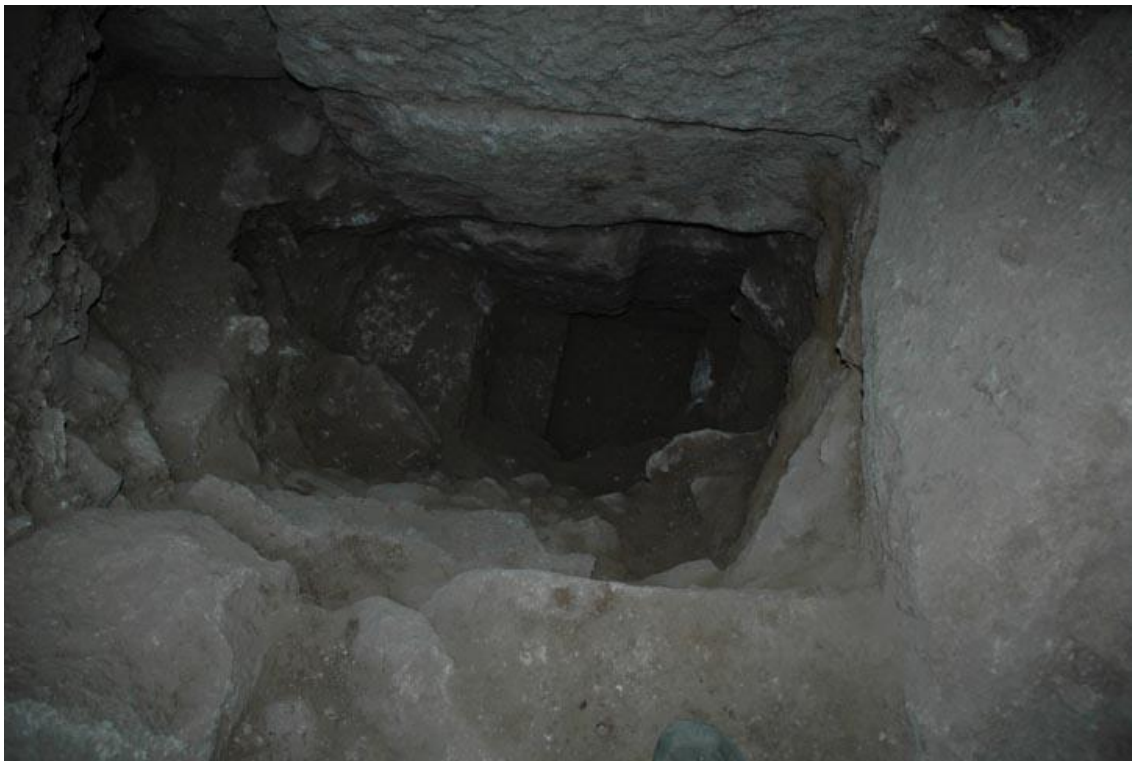
Figure 42 - The foundation investigation in front of the east wall of cella [3].
