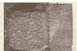
Figure 23 - A vertical lead flowing duct and a slot with one open side under the duct. Magnesia [3].
