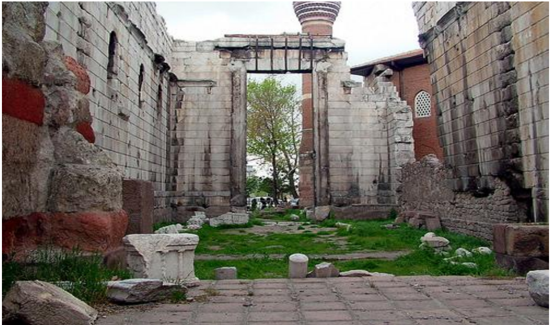
Figure 40 – Inside of cella of Augustus Temple
